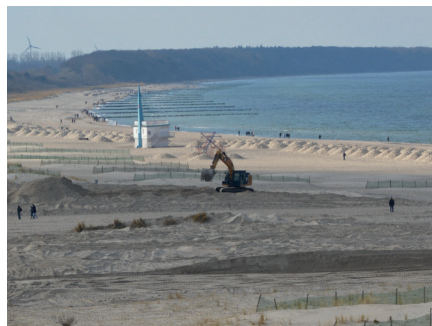
Figure 26 Sand nourishment in progress (© EUCC-D)
