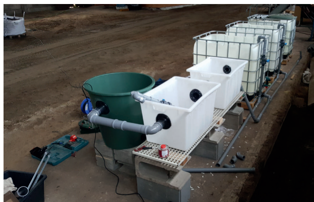
Figure 1.8 Building of the eelgrass washing unit at the Hanseatische Umwelt CAM GmbH facilities, June 2020)
